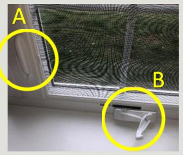
3. Push the lock (A) down while still holding onto the crank (B). (Leaving crank out)
