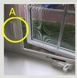
1. Be sure the lock (A) is in the up, unlocked position.
